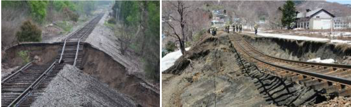
Fig. 1. Collapse of railway embankment along Plymouth Rd, Ann Arbor, US, in May 2011 after a heavy rain on already saturated ground (left); Massive landslide in Hokkaido leaves railway tracks hanging in mid-air, April 2012 (right).
