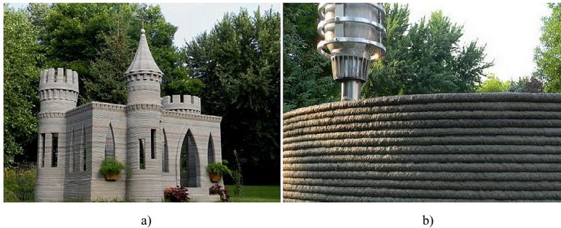
Fig. 2. (a) First structure printed in-situ; (b) printing progress [7].
