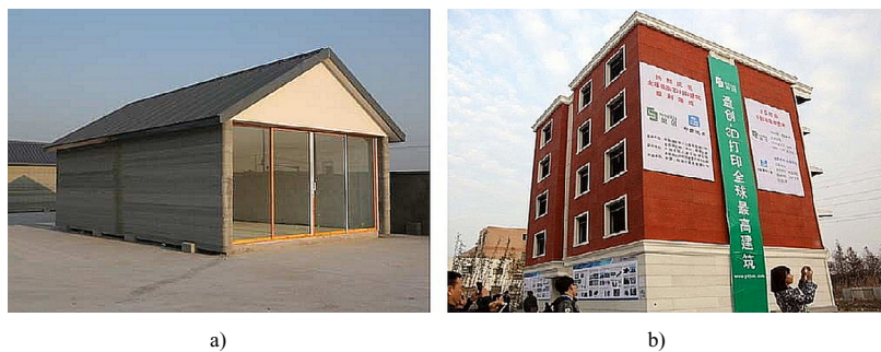
Fig. 1. (a) First house printed by a WinSun company in 2014; (b) Five-storey building printed in 3D [5].
