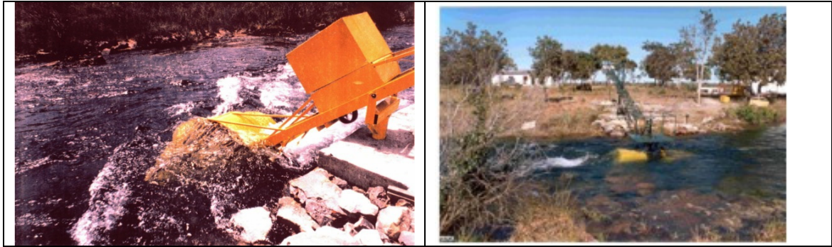
Figure 1. Hydrokinetic turbines installed in the central Brazil hinterland.
