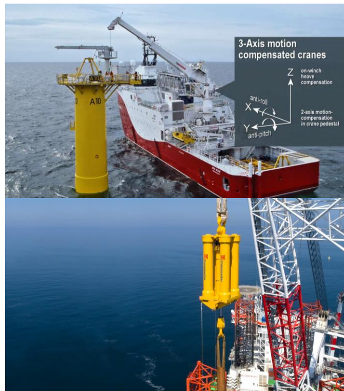
Figure 5-17: Top: SOV (vessel: Seaway Moxie) equipped with offshore crane allowing active compensation of the vessel's motion in heave, roll and pitch [Source: MacGregor]; Bottom: Illustration of auxiliary equipment for heave compensation positioned between crane hook and payload [Source: Cranemaster].
