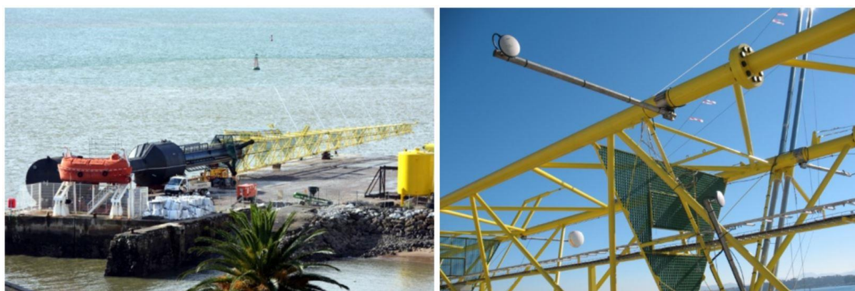
Figure 4-8. Idermar met mast [26].
