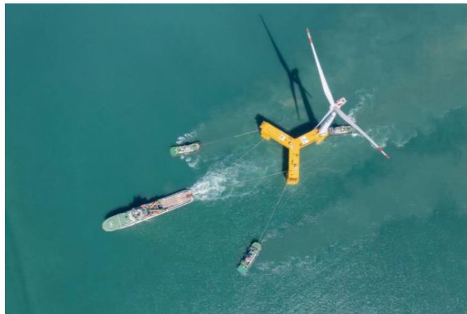
Figure 8: Sail-out of China's first FOWT off the coast of Yangjiang City, July 2021. [Source: MingYang Smart Energy]
