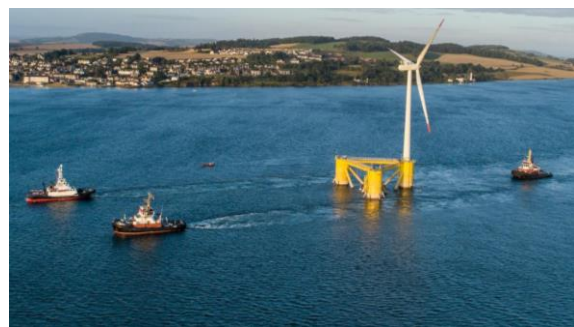
Figure 5: WindFloat semi-submersible floating offshore wind foundations at Windfloat Atlantic 2 (left) [Source: https://www.powermag.com/floating-platforms-are-an-offshore-wind-gamechanger/ ] and for Kincardine offshore wind farm (right) [Source: https://www.grupocobra.com/en/proyecto/kincardine-offshore-floating-wind-farm/ ]
