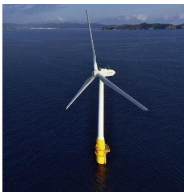
Figure 11: 2 MW FOWT on a hybrid spar foundation in Sakiyama, Japan [Source: Toda Corporation]
