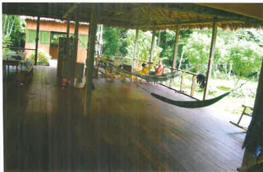
The main deck of the Las Piedras Biodiversity Station.
