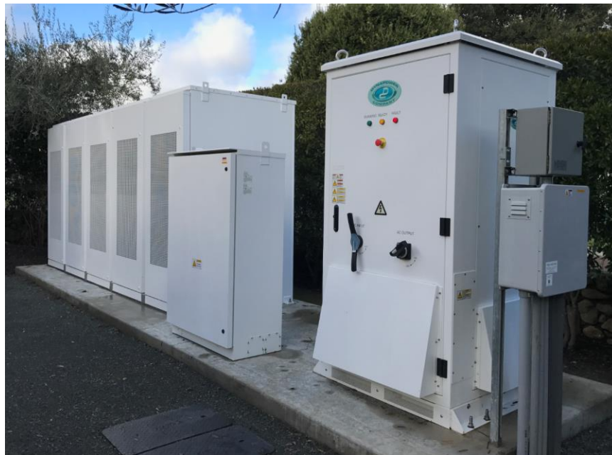
Figure 2-8: Tesla LithiumIon BS in Stone Edge Farm MES.
