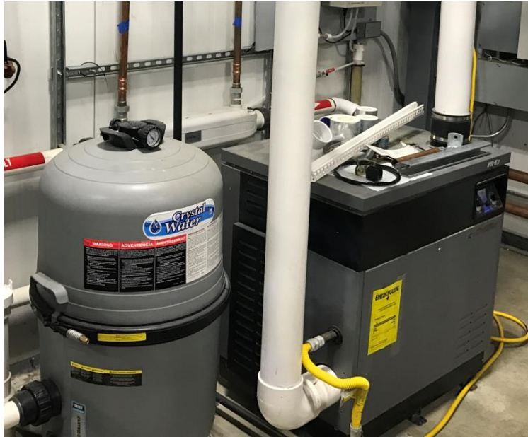
Figure 2-5: EHP in Stone Edge Farm MES.
