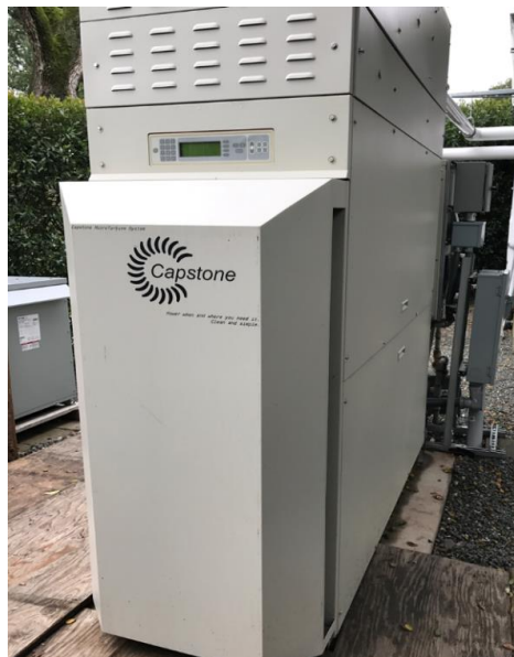
Figure 2-4: CHP in Stone Edge Farm MES.
