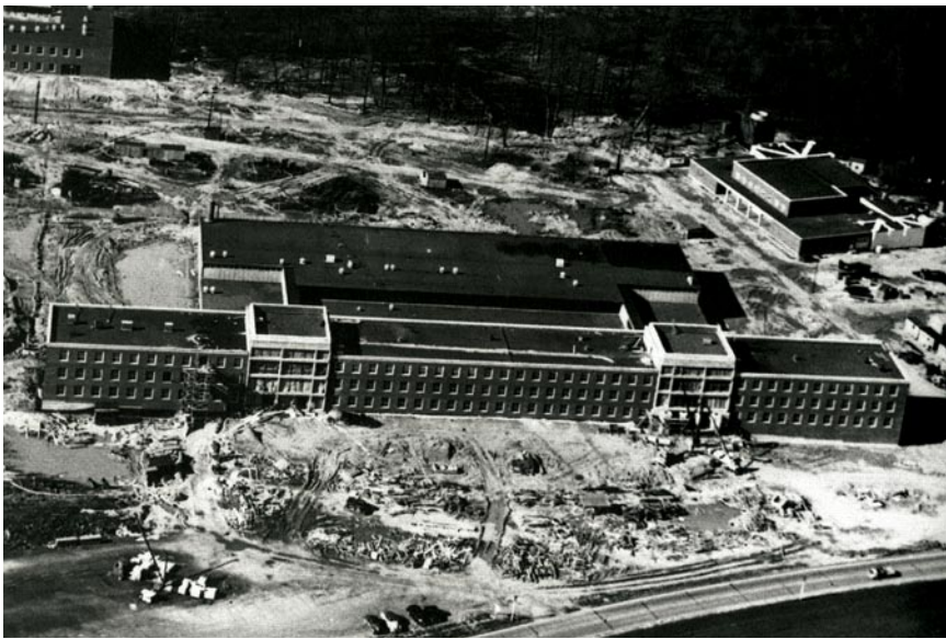
Construction of Glenn L. Martin buildings, courtesy University Archives
