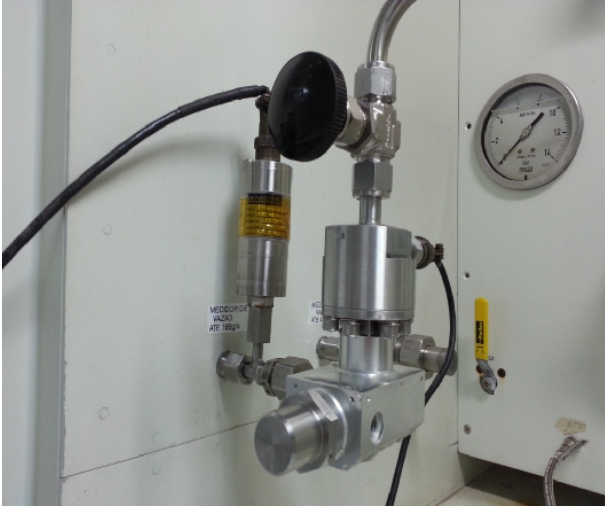
Figure 4. Gas generator valves assembly mounted for water flow test
