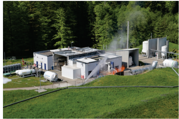
Figure 17. P8 test stand at DLR Lampoldshausen
