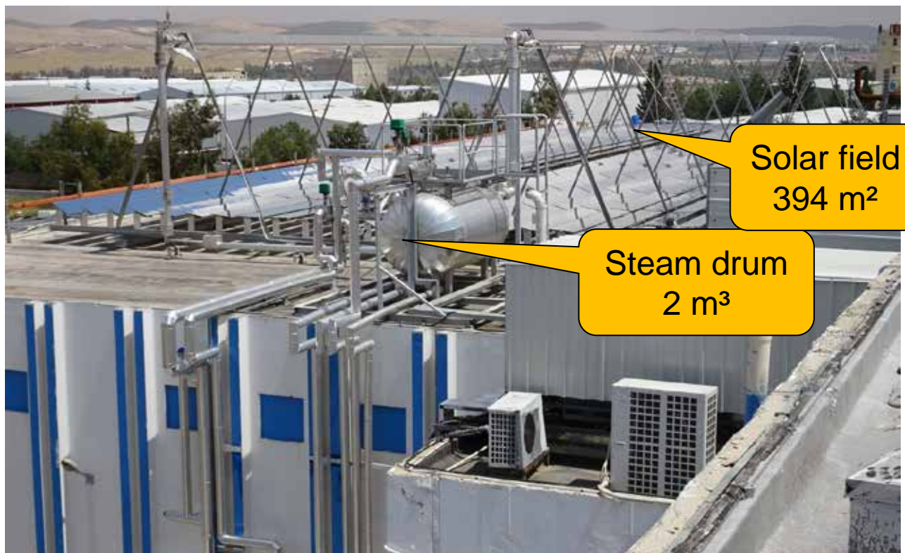
Collector field and steam drum with piping to steam network
