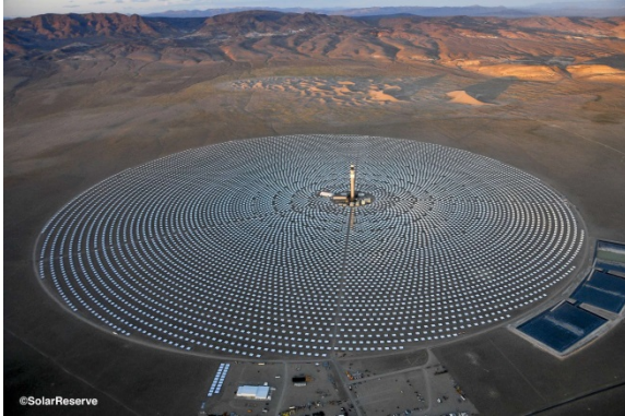
Reference system: molten salt, steam cycle @540°C
