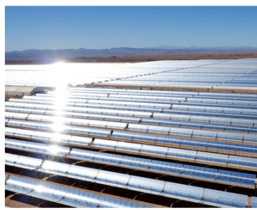
Abbildung 1-3: Parabolrinnen-Anlage (Quelle: Centrale Solaire Noor owned by masen © Ciments du Maroc)
