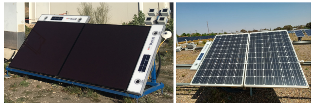
FIG. 1. Measurement setup. Left picture (at CIEMAT's PSA) - Fixed PVRC and DustIQ's installed with a tilt of 45^\circ facing south. Right picture (at IRESEN's GEP) - Two solar modules and DustIQ mounted with a tilt of 30^\circ facing south.
