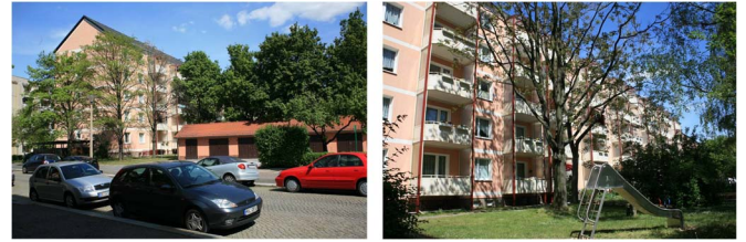
Fig. 4. Optical image of building. (Left) View from the side. (Right) View from the front (copyright G. S.).
