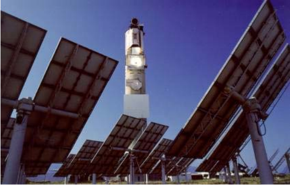
Solar thermal power plants
