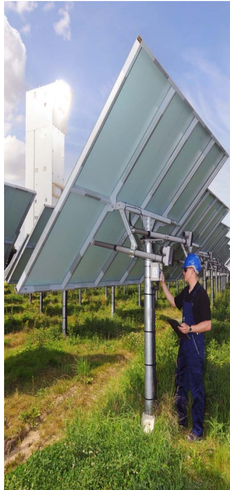
Solar Power Tower
