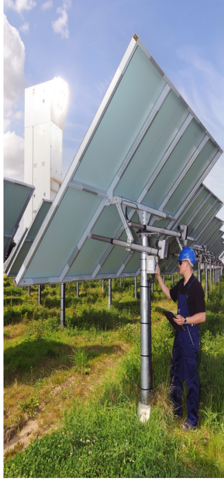
Solar Power Tower
