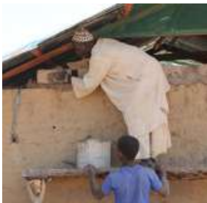
Closing Eave Gaps in the Gambia. Credit: Steve Lindsay
