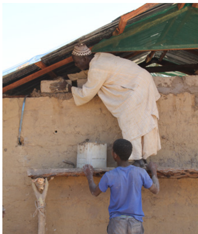
Closing eave gaps. Photographed by Steven Lindsay.
