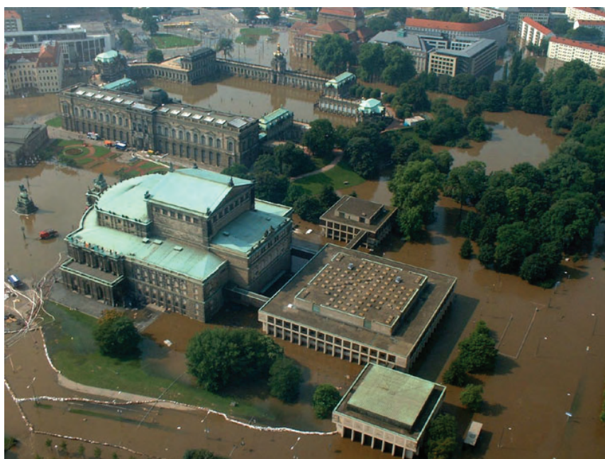
Figure 1: Flood in Dresden in 2002, Semper Opera (courtesy: Feuerwehr Dresden).
