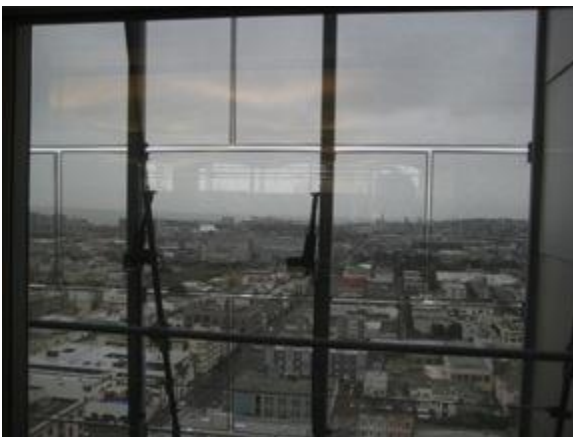
Fig. 3. Interior view looking out through SE facade glazing, retrofit solar control film, and exterior perforated metal panels (with interior roller shades retracted).
