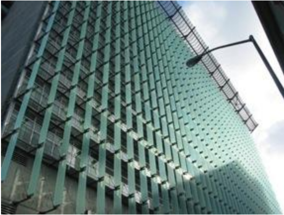
Fig. 5. Exterior view of the NW facade showing fixed exterior translucent vertical fins [16].
