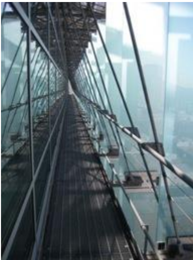
Fig. 6. View from catwalk within NW facade showing exterior vertical translucent fin shading devices. The partially transparent optical properties of the fins can be seen towards the bottom right of the image.
