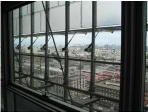
Fig. 3. Interior view looking out through SE facade glazing, retrofit solar control film, and exterior perforated metal panels (with interior roller shades retracted).
