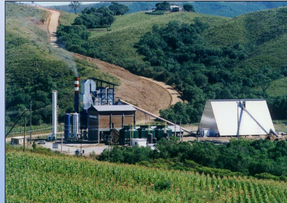
Wood residues power plant, 10 MW Piratini, RS Brazil
