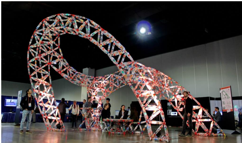
Figure 4: TrussFab pavilion created from ~1200 PET bottles and 119 3D printed hubs, presented at CHI'17, Denver, USA.
