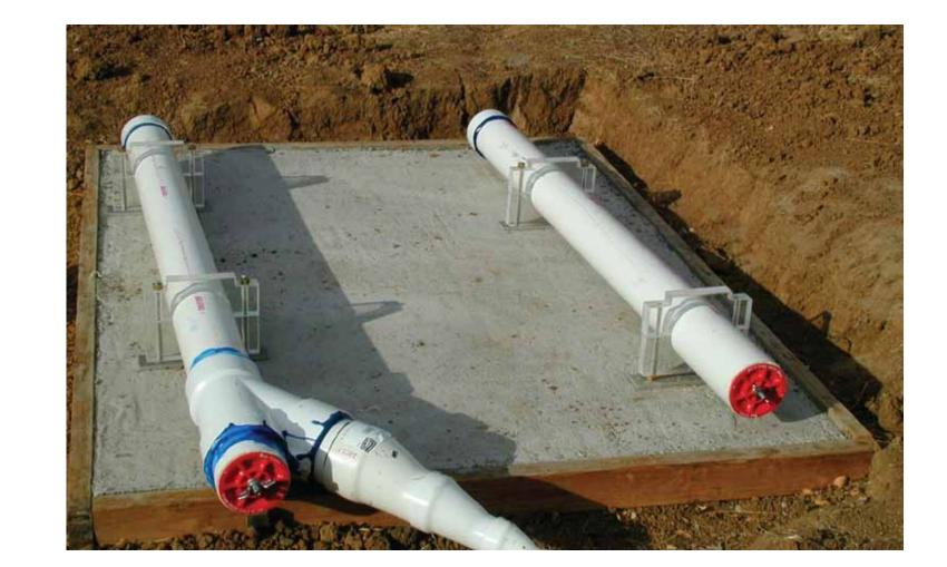
Photo of new, unburied coil housing. Each site will have a duplicate, parallel PVC housing for testing purposes.
