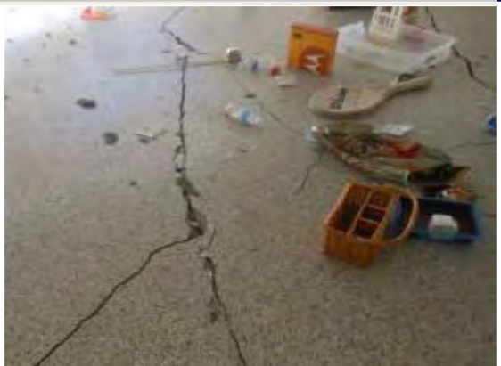
Cracked garage slab
