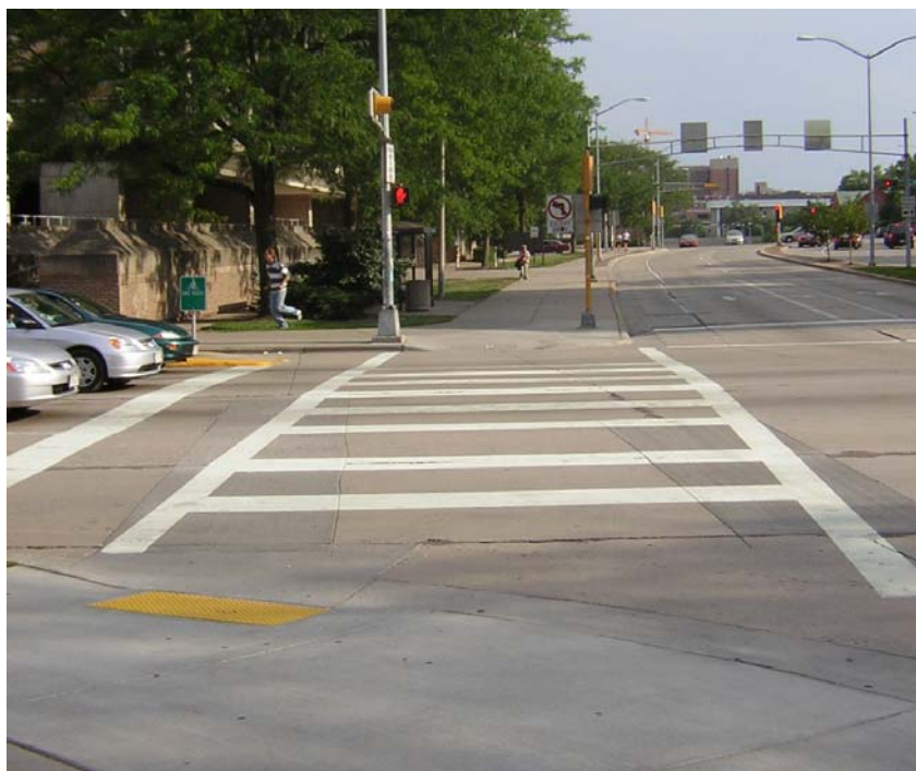
FIGURE 1 Signalized crosswalk at Park St. crossing University Ave. in Madison, WI.
