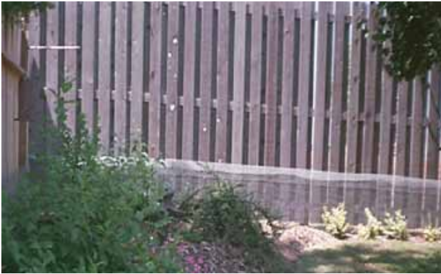
Figure 5. A rabbit fence added to an existing fence.
