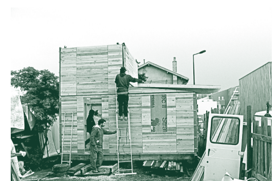
Low-cost house from scrap timber © Bois & Cie
