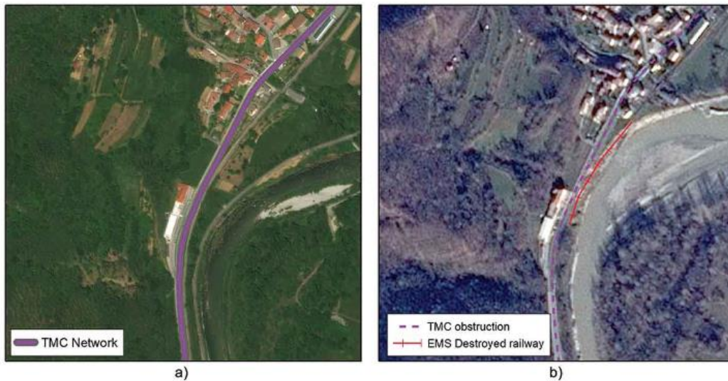
Figure 99: Damages to the transport network. (a) shows the pre-event situation. (b) shows how EMS-Mapping reported damages only to the railway network while TMC reported an obstruction event to the nearby road too.
