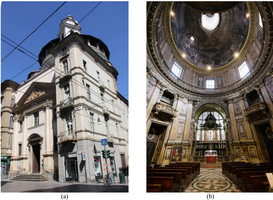
Figure 1: The SS. Trinità church in Torino: (a) outside view; (b) inside view.
