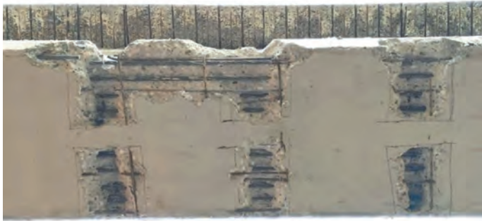
Figure 3. Strands cutting in B5-P46/47 girder (bottom view).
