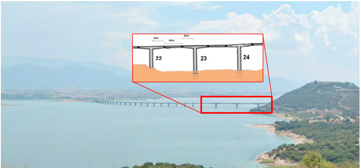
Fig. 1. General view of the Polyfytos lake and the bridge with the detail of Piers #22, #23, #24.
