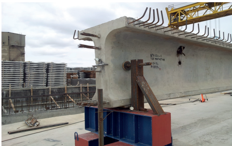
Figure 17 The support zone of the VTK-33u beam with dial indicators
