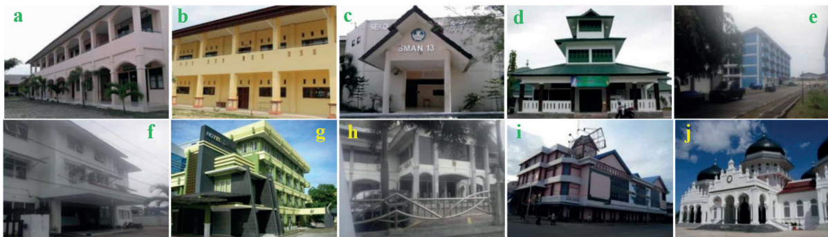
Figure 4 (a) Public Elementary School 70 (SD), (b) Public Junior High School 12 (SMP), (c) Public Senior High School 13 (SMA), (d) Tgk. Dianjong Mosque, (e) Low-cost Rental Apartments, (f) Cut Mutia Hospital, (g) Hotel Lading, (h) State Electricity Company, (i) Pasar Aceh Building, (j) Baiturrahman Mosque
