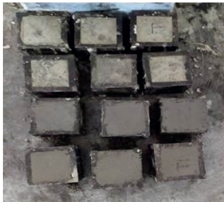
(a) Casting Concrete
