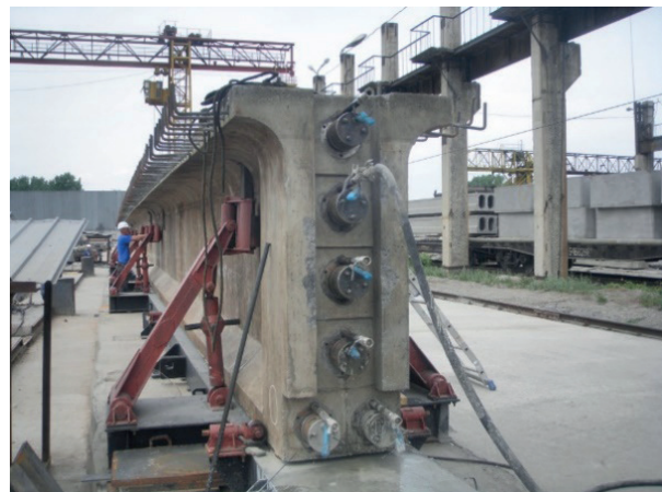
Figure 9 Injection of cement grout into the second duct
