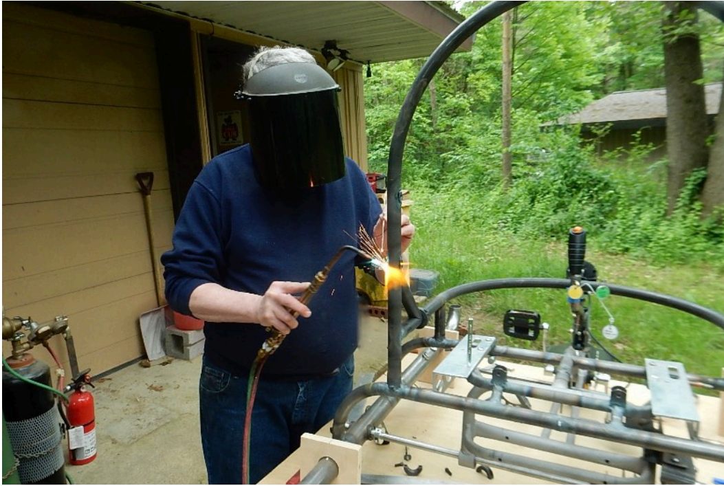
Tack welding braces to strengthen the tube structure.
