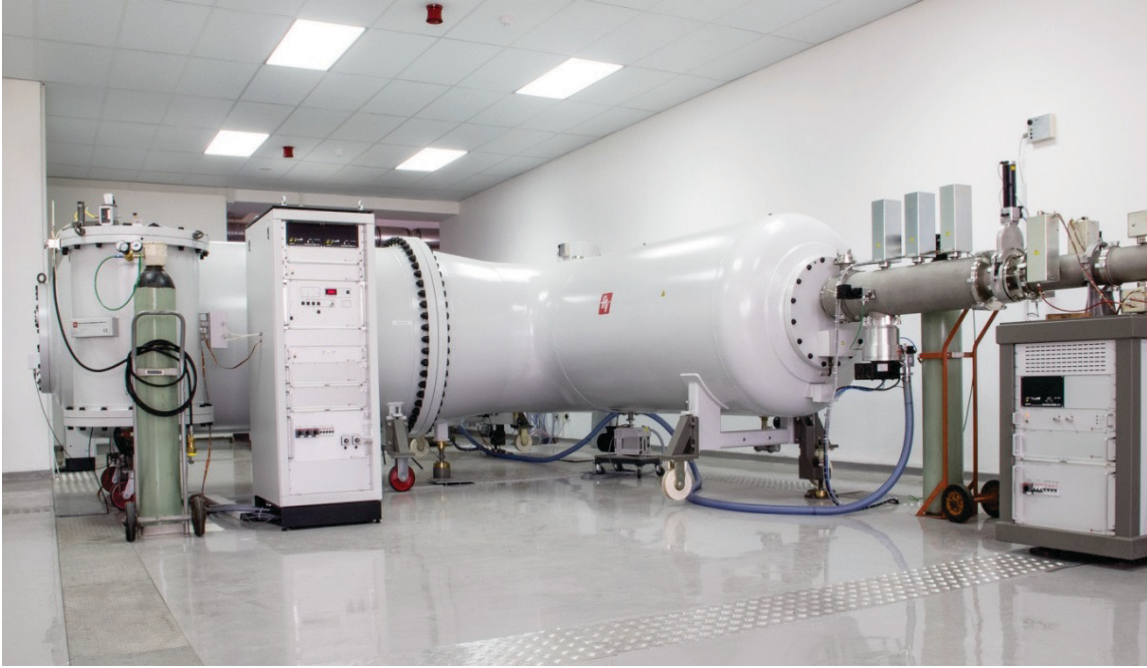
Figure 1: New 3 MV Tandatron Accelerator for the Materials Research Department (MRD).
