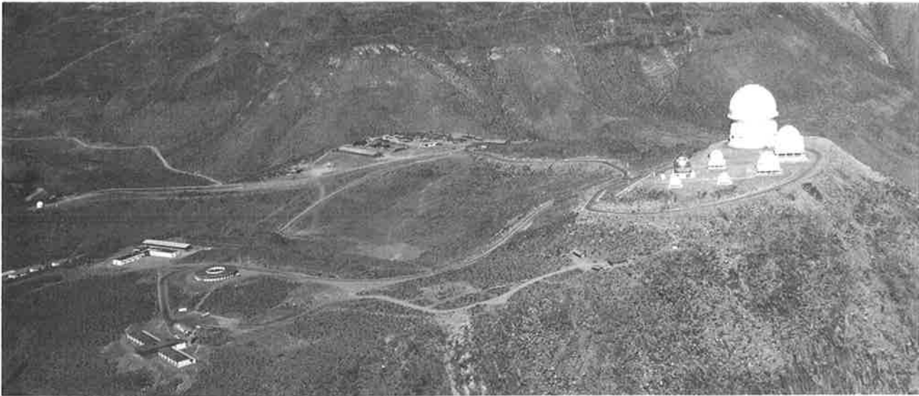
Primary facilities of the Cerro Tololo Inter-American Observatory are located at an altitude of 7,200 feet in the Chilean Andes. Among the stellar telescopes at the right is the largest telescope (4-meter) in the Southern Hemisphere, which was brought to operation during fiscal year 1975. Visiting scientists' quarters, laboratories, and support facilities are at the lower left. [Photo by Kitt Peak National Observatory]
