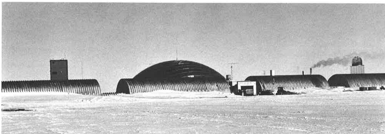
The new Amundsen-Scott Pole Station, with its 164-foot diameter, 50-foot high geodesic dome and arched structures for scientific research, was dedicated January 1975.
