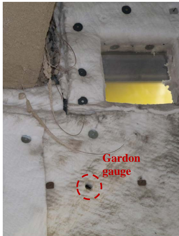
Figure 4-7 Gardon gauge mounted on the east wall.
