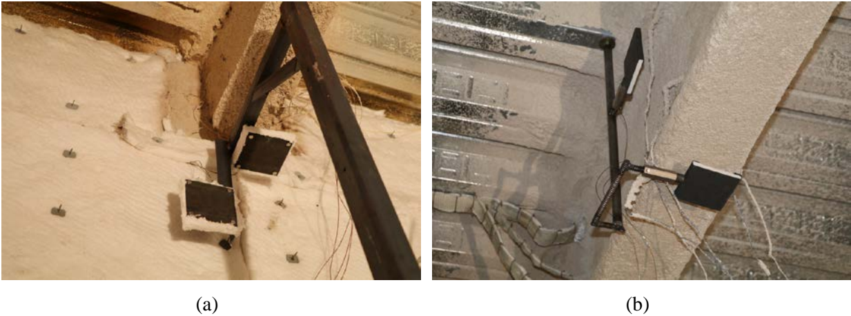
Figure 4-8 Location of plate thermometers: (a) east connection; (b) mid-span of the beam.
