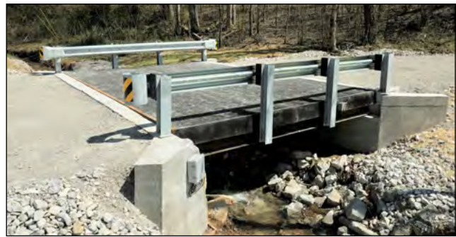
Fiber-Reinforced Polymer Vehicle Deck Bridge. Credit: IACMI
