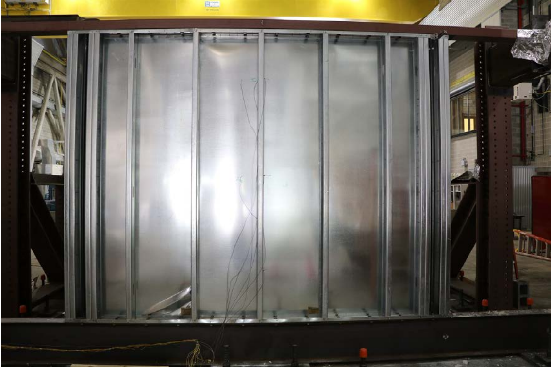
Figure 48: CFS01 - Photograph of back of metal sheathed side of wall after mechanical loading; nonstructural gypsum removed.
