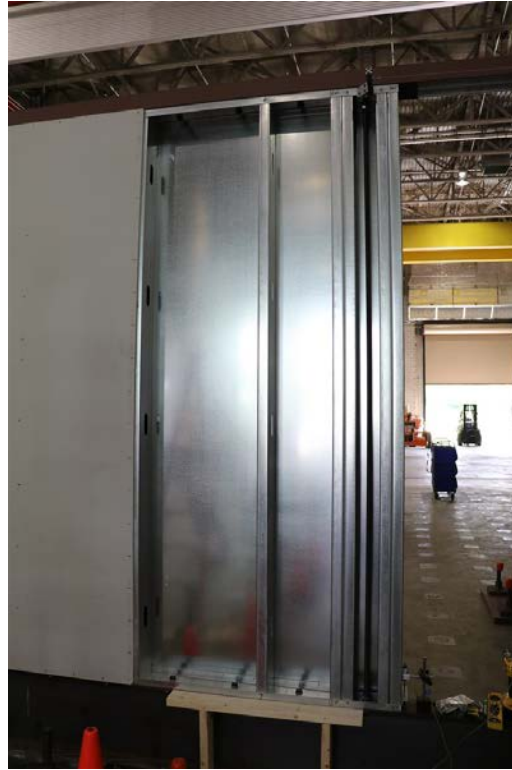
Figure 6: Photograph of test specimen with one gypsum board removed.
