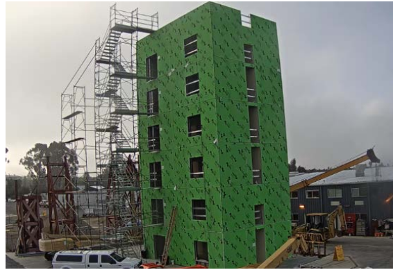
Figure 1: Cold-formed steel framed building at the UCSD test facility.
