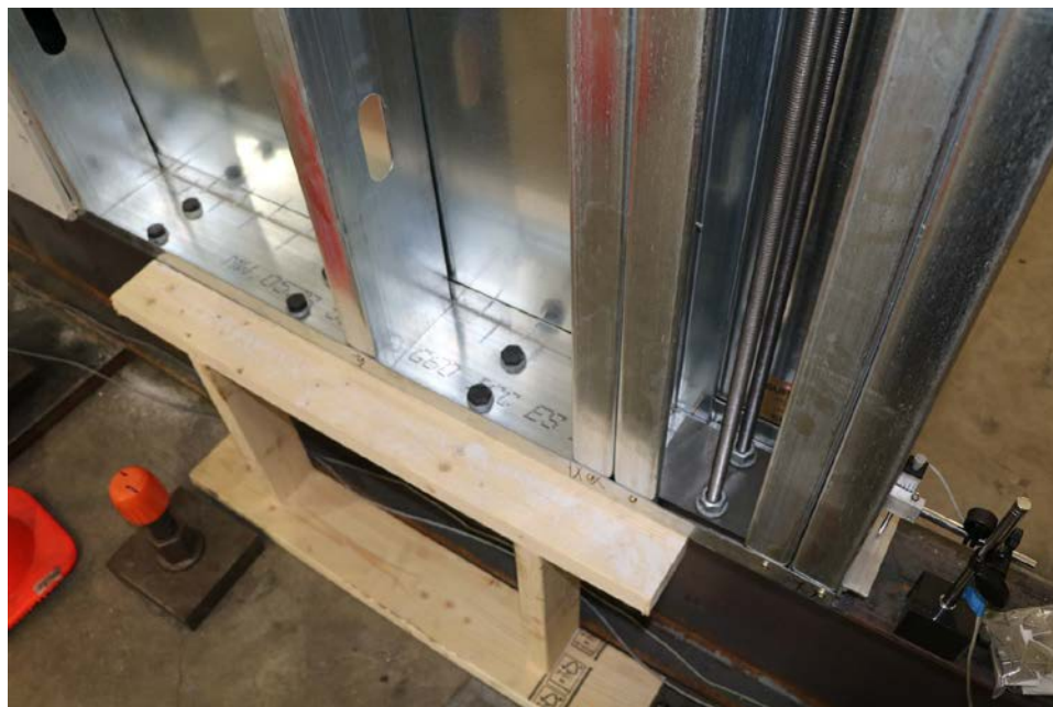
Figure 15: Photograph of plate washer on bottom of tension tie rods.
