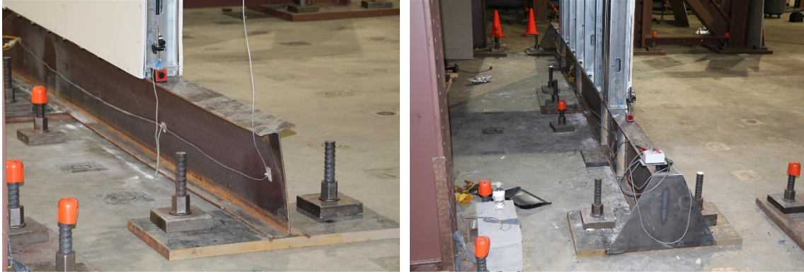
Figure 45: CFS01 - Photograph of bottom framing beam: (a) during test; (b) retrofit for all subsequent tests.
