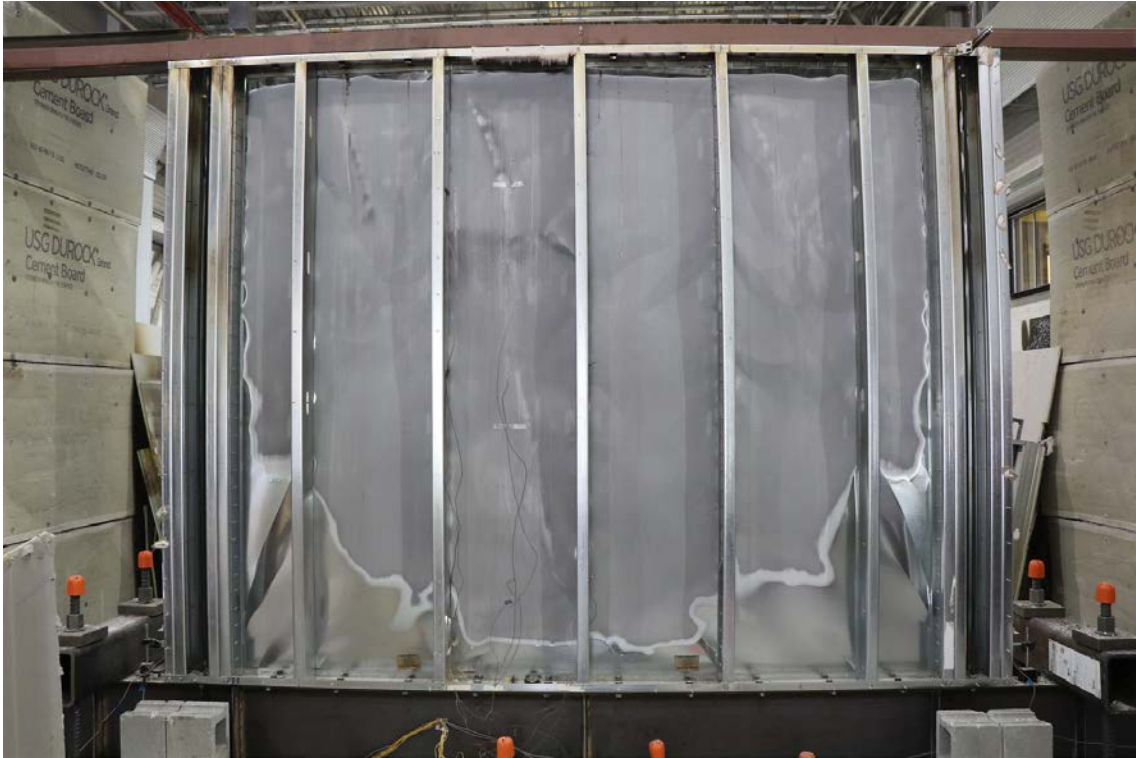
Figure 104: CFS06 – Photograph of back of metal sheathed side of the burned wall after mechanical loading to 2.8 % drift (CFS06c); nonstructural gypsum removed.
