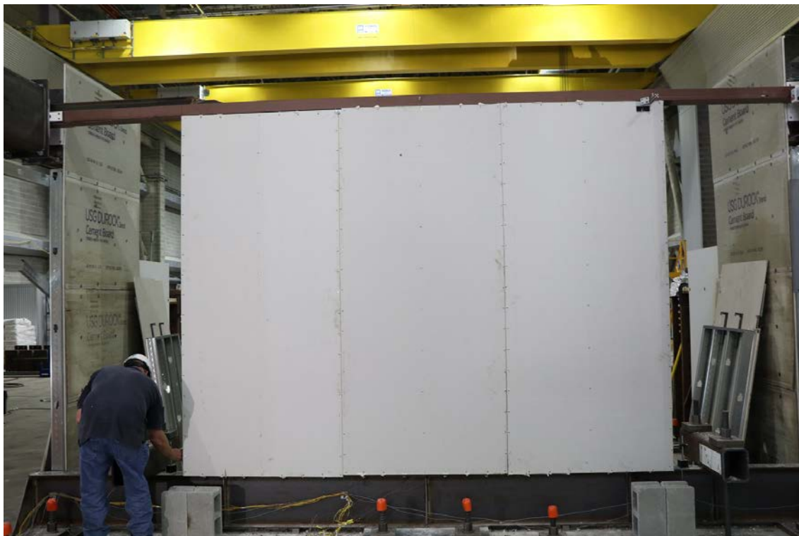
Figure 70: CFS03 – Photograph of gypsum sheathed side of wall after mechanical loading to 2.8 % drift (CFS03c).
