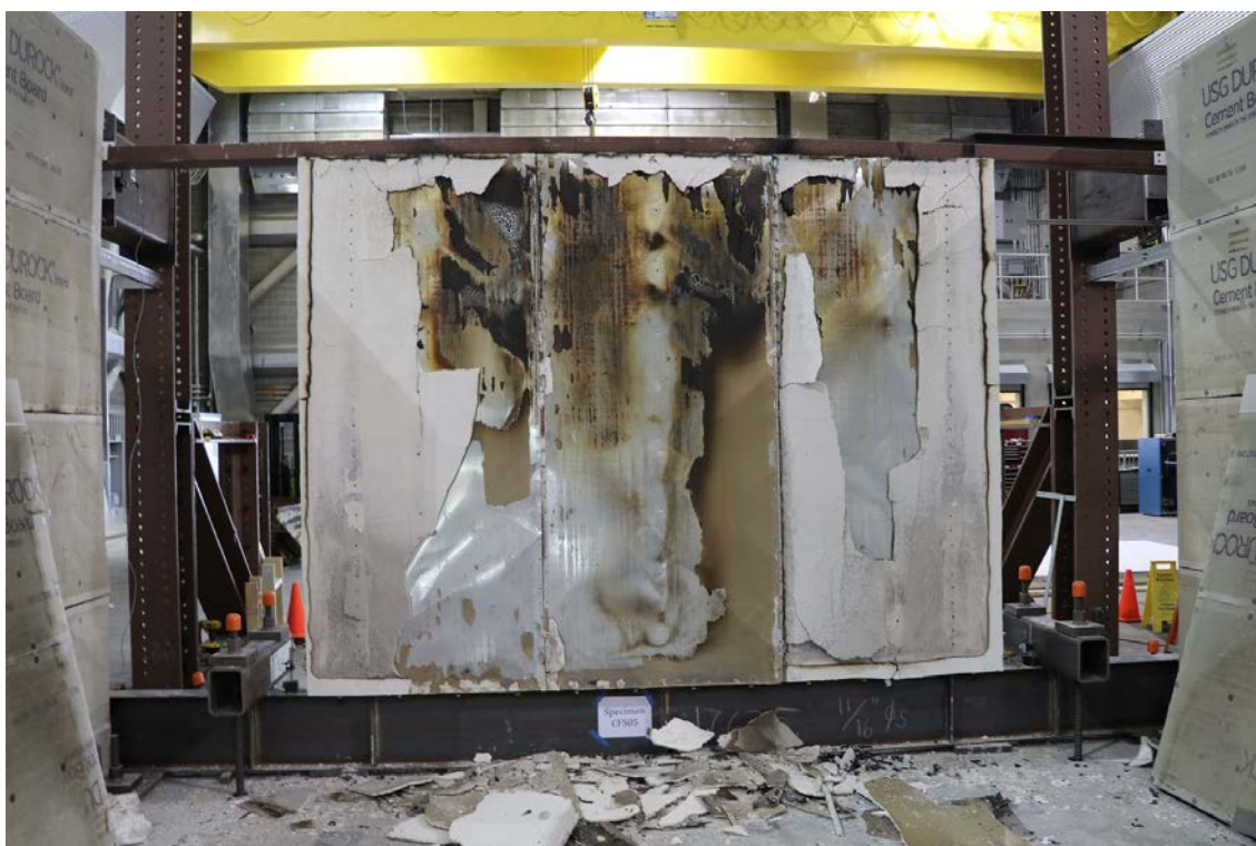
Figure 92: CFS05 - Photograph of metal sheathed side of the burned wall after mechanical loading to 2.8 % drift (CFS05b).
