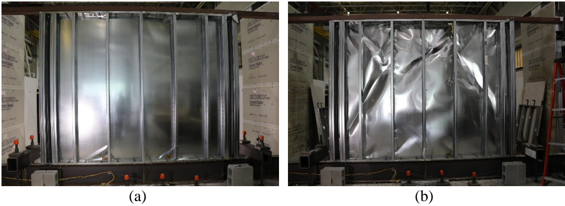
Figure 30: Photograph of back of metal sheathed side of wall after mechanical loading to 2.8 % drift; nonstructural gypsum removed: (a) unburned wall; (b) wall after burning.
