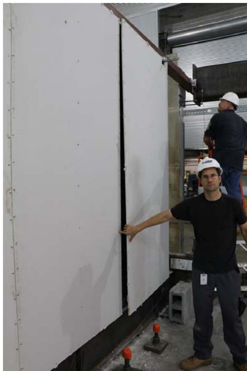
Figure 72: CFS03 – Photograph of gypsum sheathed side of wall after mechanical loading to 2.8 % drift (CFS03c) highlighting board detachment.
