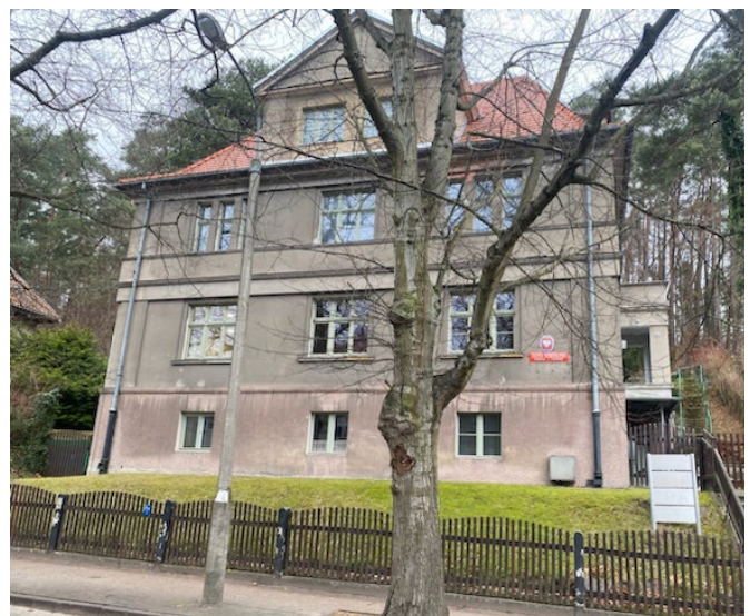
The villa at Antoniego Abrahama Street. Credit: IM PAN.
