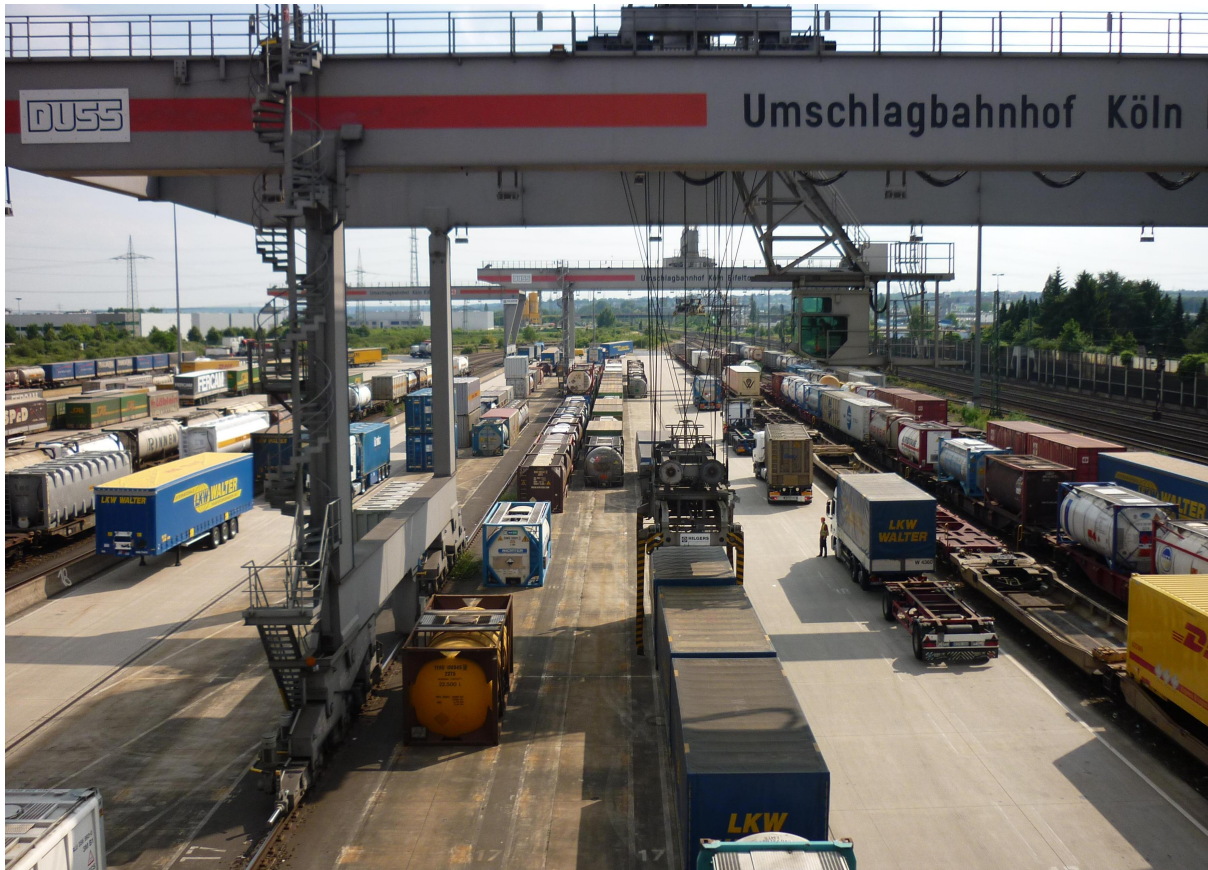
Figure 2.2: This picture shows a rail-road terminal (Köln Eifeltor) with rail, road and storage areas and overspanning cranes.
