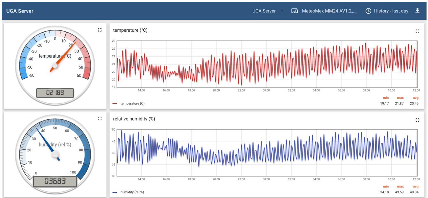
Figure 8 Monitoring the air conditioning of a high-performance computing server room.
