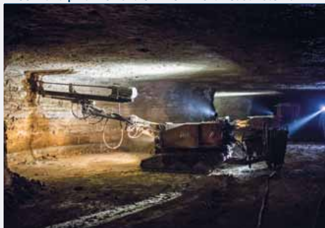
EESTI ENERGIA operates one underground and one opencast mine as well as a rail transport division
