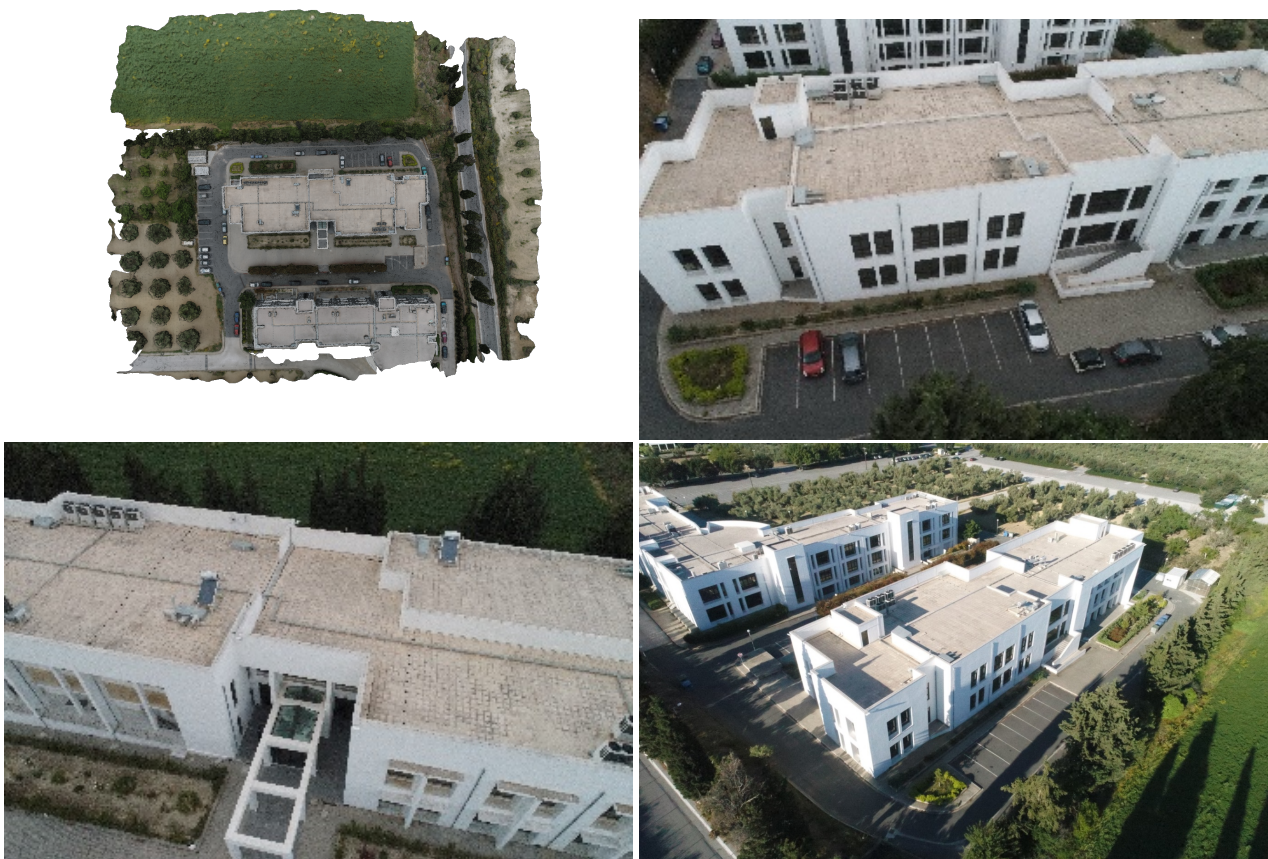
Figure 4. Top and side views from outdoor reconstruction of a building using aerial photogrammetry.
