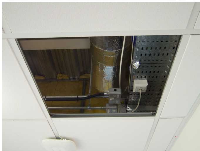
Figure 4.47: Metalwork abundant in department building ceiling.
