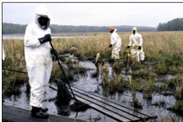
Figure 3-5. Workers using snares on poles to remove thick oil floating on the water surface deep in the brackish marsh interior at the Chalk Point oil spill on the Patuxent River, Maryland in April 2000. Note the use of walking boards. Photo credit: Jacqueline Michel.
