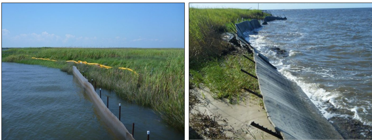
Figure 3-3. Shoreline barriers used during the Deepwater Horizon oil spill. Filter fences require many steel posts to keep them in place. Usually there is not enough time to deploy this type of barrier after a spill, they have limited effectiveness, and are difficult to remove. Also note the hard boom stranded on the marsh at left. Photo credit: Helen Chapman (left); Thomas Minter (right).
