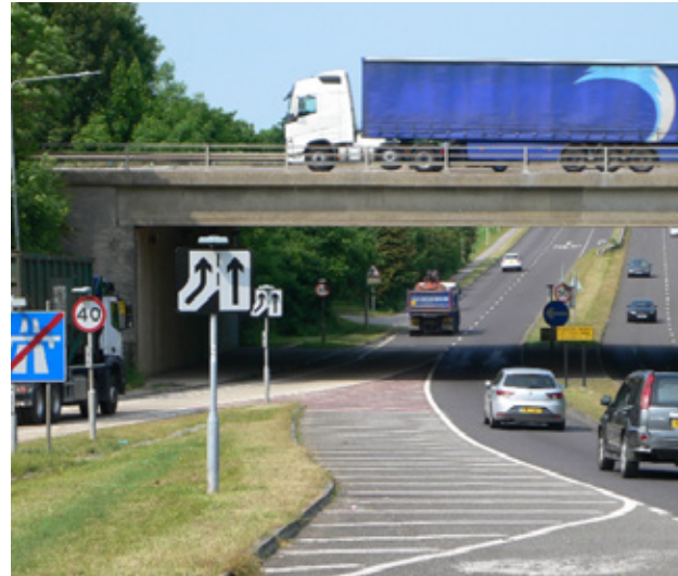
M27 junction 10 and the north going A32, near Fareham. Traffic on the A32 has been moved to the outer lane to provide a protected entry lane for merging traffic.
