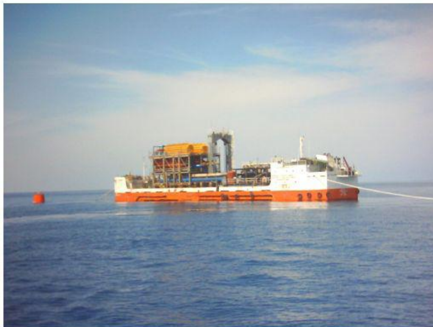
Figure 3.7: A View of the Barge-Mounted Desalination Plant
