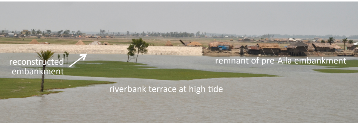
Figure S9 | Field photos showing embankments and repair efforts on Polder 32. a , Local and regional labor reconstructing a portion of embankment. Concrete blocks are made on site and emplaced by hand. Embankment repair and maintenance was an important income source following Cyclone Aila during the temporary loss of local livelihoods such as shrimping and rice cultivation. Photos taken at low tide. b , Repaired sections of the Polder 32 embankment observed along the Sibsa River during high tide.
