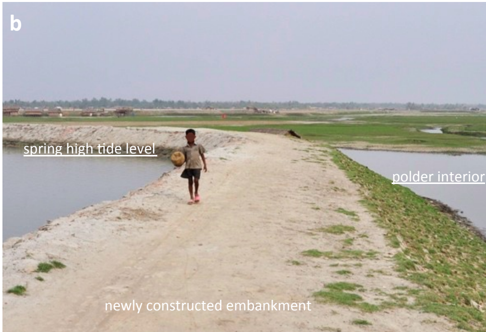
Figure S6 | Field photos contrasting tidal channel water levels with Polder 32 interior. a, b Photos of newly reconstructed embankment along one of the major breaches. Images taken near to spring high tide, contrasting the relative elevation between high water and the polder interior.
