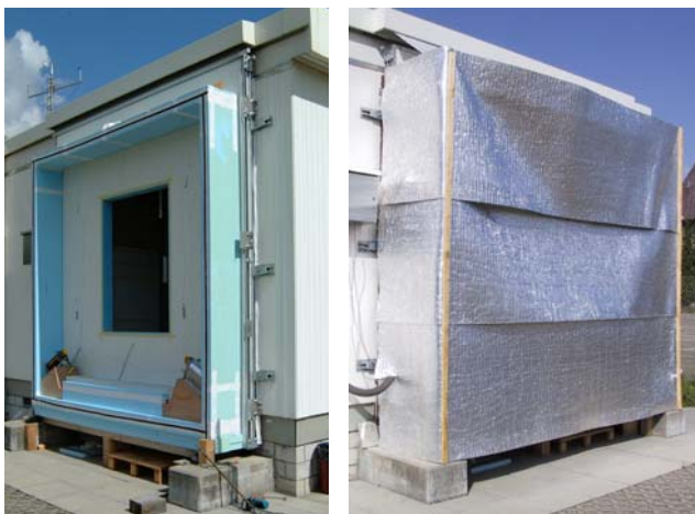
Fig. 3 Thermally controlled external chamber mounted in front of one of the cells and viewed from outside during (left) and after construction (right).
